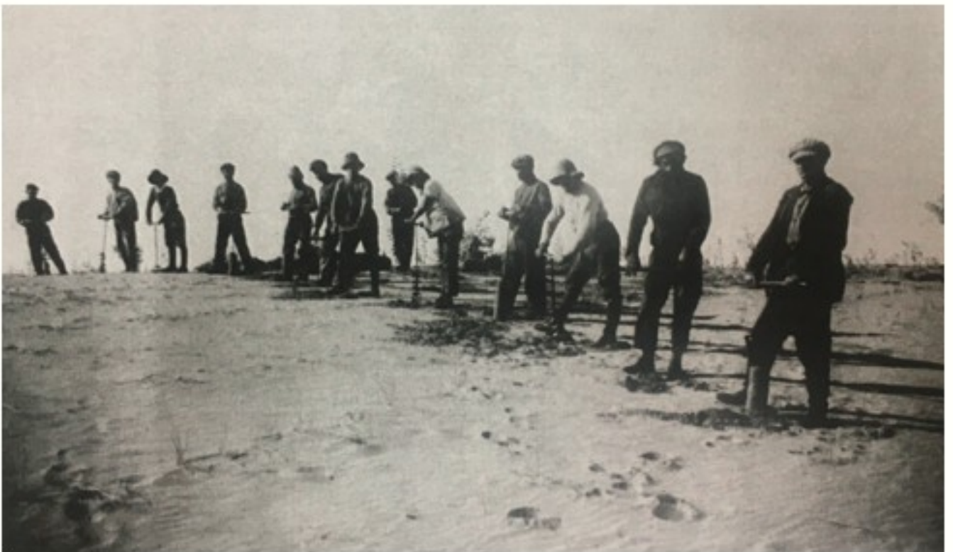
Elders are mobilized to plant trees on the land of newly independent Israel.
